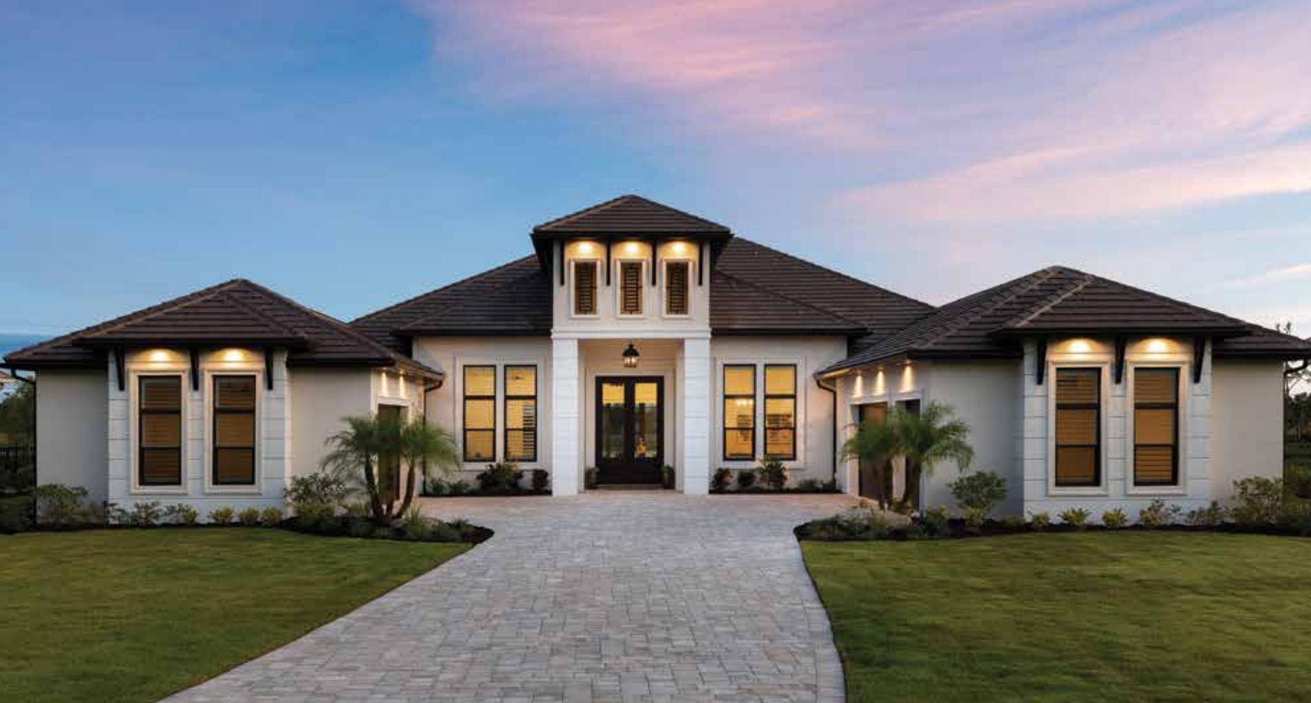
Above: Clean lines characterize the contemporary exterior. Iron corbels custom-designed by Johnson support the roof and its chocolate-brown concrete tiles. White stucco in a shiplap-like design brightens the home's façade. The contrasting light and dark finishes of the exterior are indicative of the sophisticated scheme that lies within.
